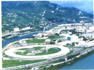
The European Synchrotron Radiation Facility in Grenoble, France. Compound refractive lenses may soon make its intense X-ray beams much more effective.
